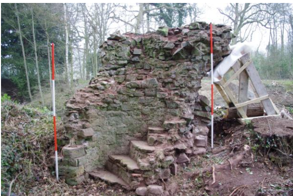
Standing remains of Bronsil Castle undergoing repair and recording. © Herefordshire Council
