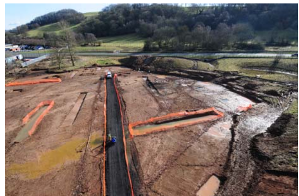
Futures site under excavation
