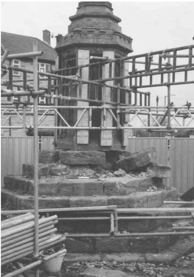
Damage to the Whitecross monument, Hereford
