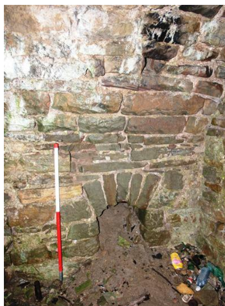
Draw arch of Whitchurch limekiln
