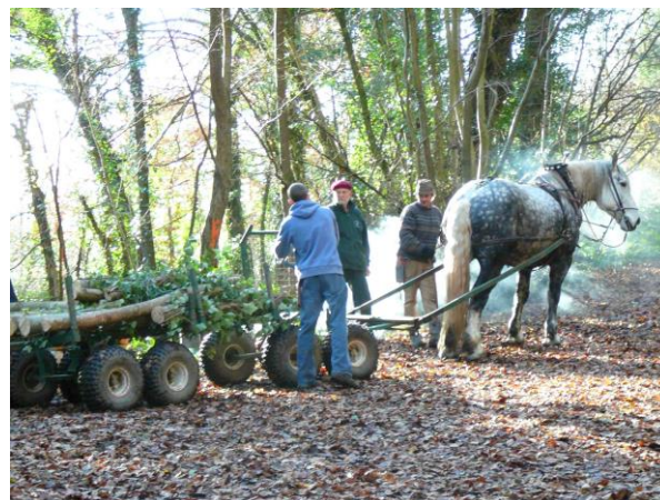
Doug Joiner's Heavy Horse team at work removing trees from the New Weir Ironworks site © Kate Biggs
