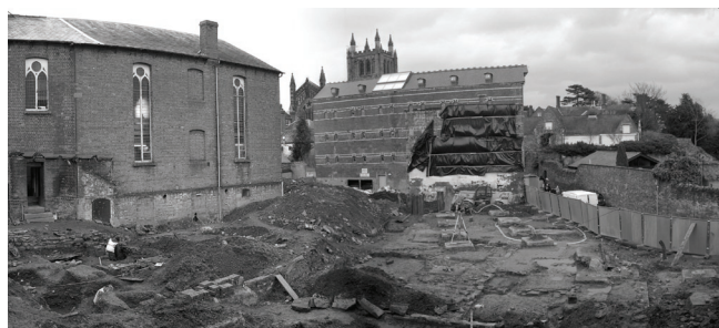
Looking west across the Crystal Rooms site
