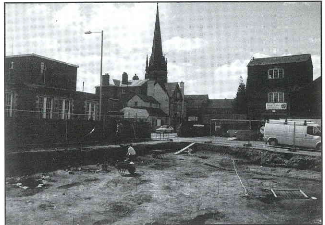
Excavations in progress at the Gaul Street site
