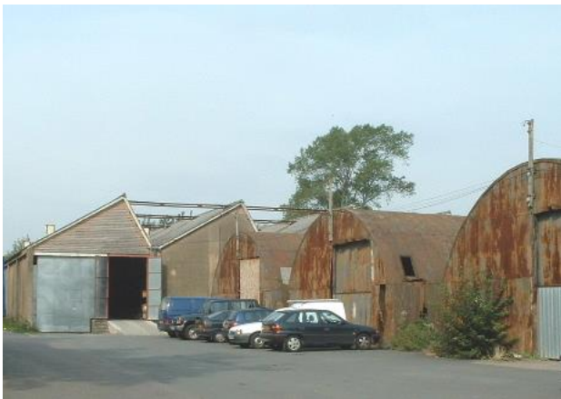
Some of the munitions buildings remain in use at Rotherwas
