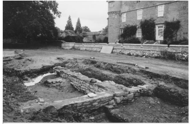
Excavations at Croft Castle reveal the buried remains of earlier buildings below the west lawn
