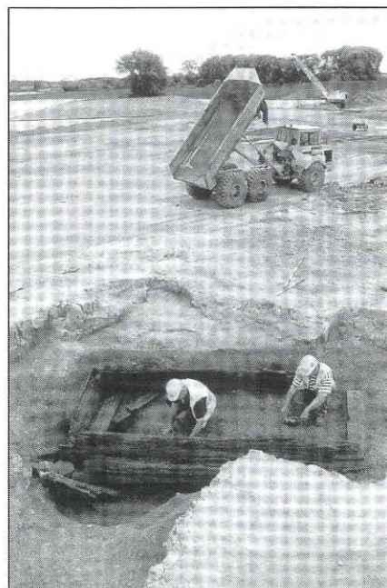
The well-preserved timber structure of a medieval watermill is uncovered at Wellington Quarry.
