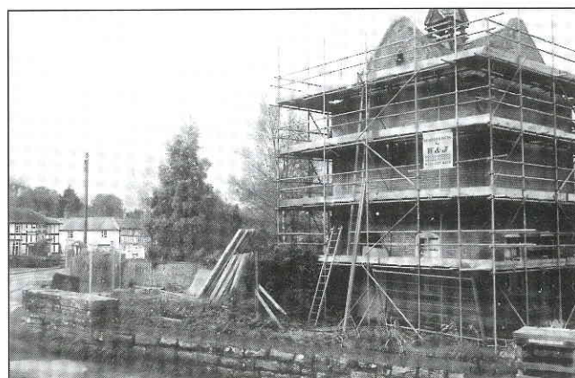
Eardisland dovecote currently being 'conservatively repaired'
