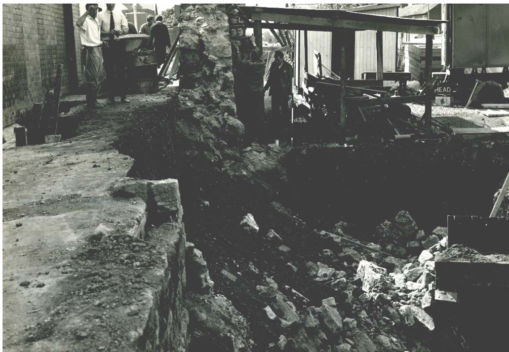
The north end of the Gunners Lane wall in 1968 following the collapse of masonry into the underpass excavations alongside (Contract photographs file, Hereford City Council)
