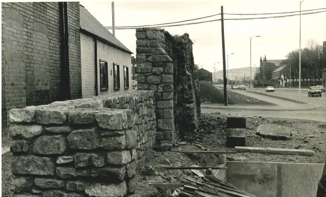
The north end of the Gunners Lane wall in April 1969 after reconstruction. Other photographs show the stones of the buttress (mid-foreground) numbered for dismantling (Contract photographs file, Hereford City Council)
