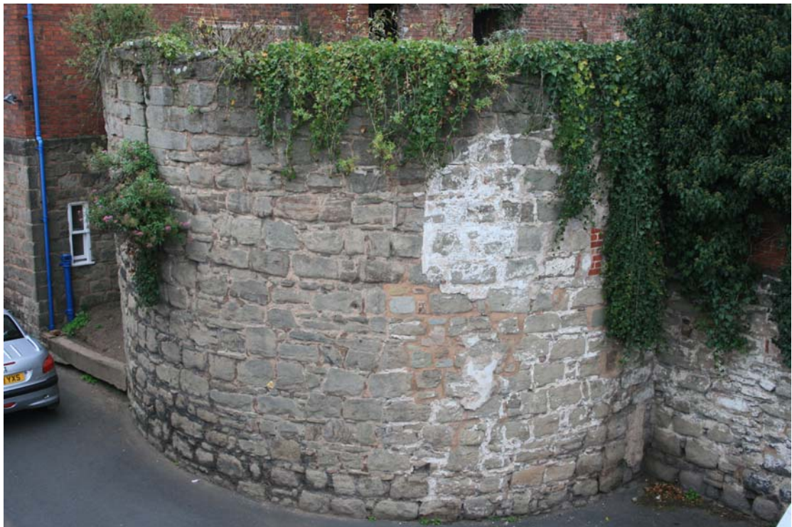
Bastion 2, adjoining the south side of the Greyfriars Surgery. The large ivy mat (right) is problematic, potentially concealing loosened masonry.
