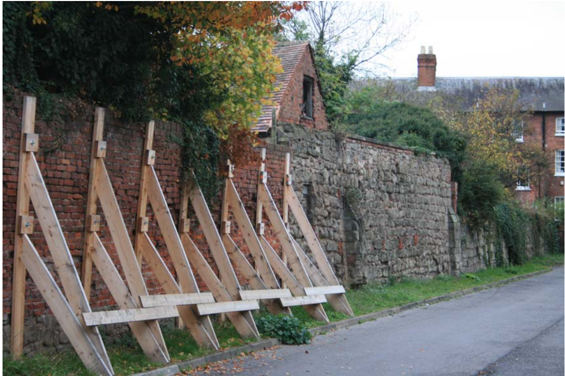
The failed brickwork stretch of wall immediately north of the Black Lion plot
