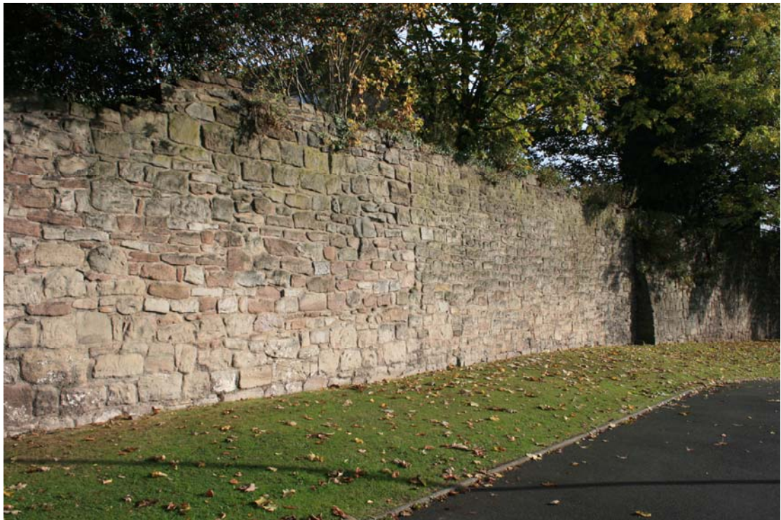
Different builds in the masonry of section 3 on the exterior face of the Berrington Street Job Centre stretch
