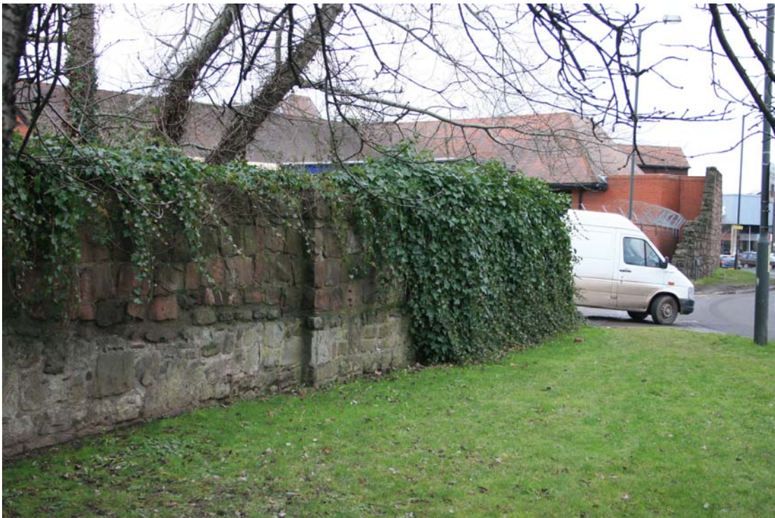
Looking west towards the north-east end of the section 7 (1968) wall beyond the Tesco vehicle exit. The section 8 wall in the foreground consists of (probably rebuilt) city wall masonry raised by the addition of the distinctive red 1968 masonry
