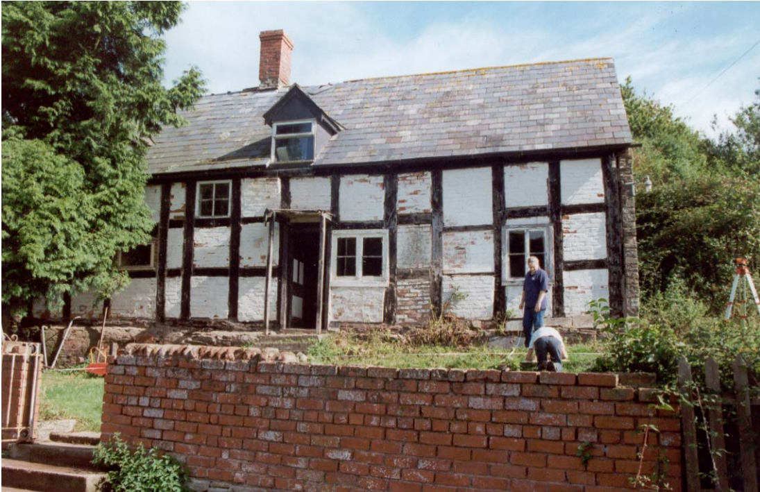
Figure 5: Photograph of Great Walk Mill Farm at the time of the survey, looking north.
